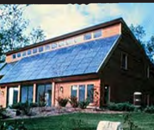
Carslile Solar House
